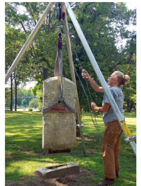
Above: Ta Mara Conde of Historic Gravestone Services demonstrates how to properly use a small tripod to lift small gravestone monuments for minor repairs.
