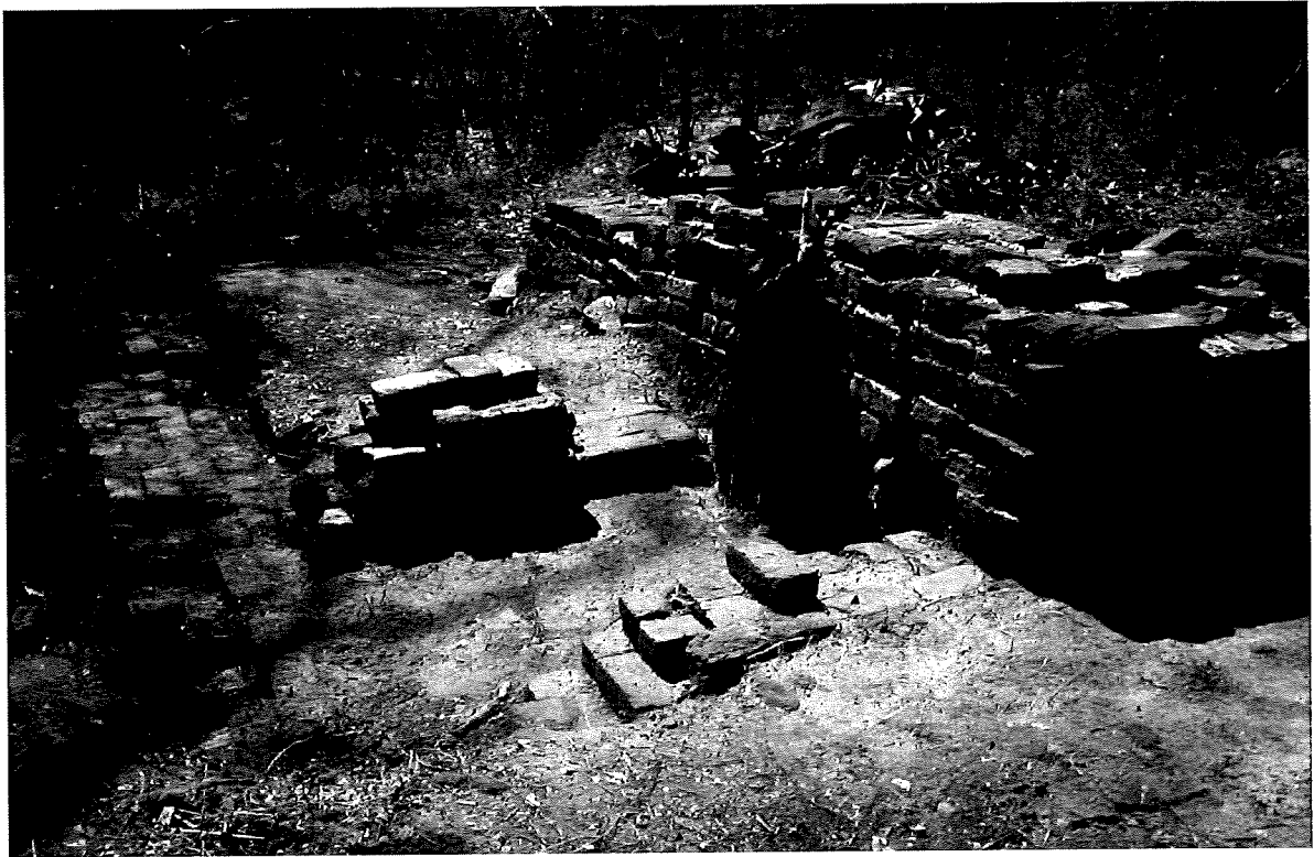
Figure 15. View of brick ruin (right) superimposed on an earlier brick foundation (left). Note large tree stump between the two. View looking southwest.
