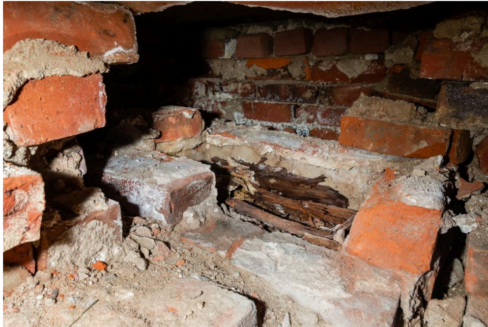
Figure 2. The interior vault with the upper course of bricks partially removed to facilitate access. Degraded pieces of lid and side panels of a wooden box are visible.
